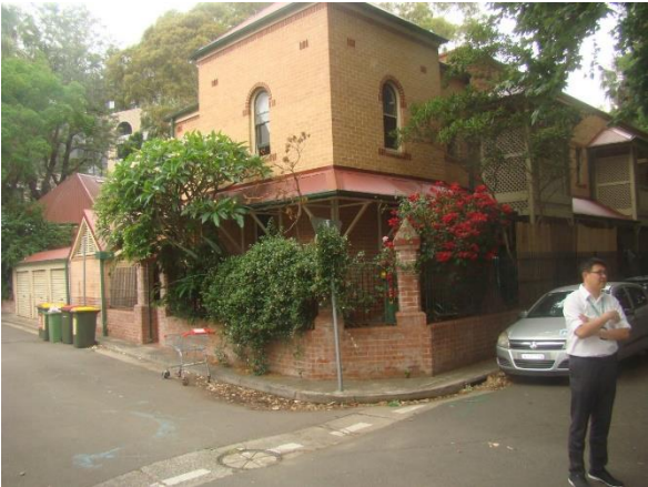
Figure 14. Corner of Wentworth Street and Cowper Street.
