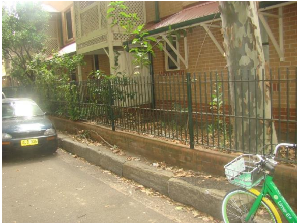
Figure 17. Sandstone kerbing along Mitchell Lane East.
