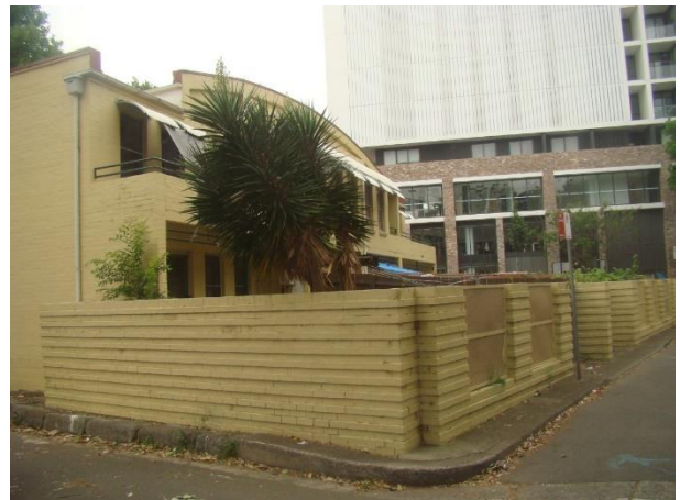
Figure 24. Rear of 2A-2D Wentworth Park Road.
